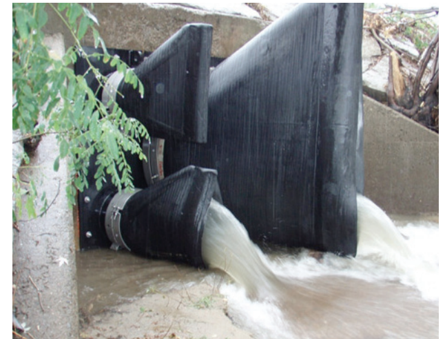
FEMA-funded valves & pumps control flooding in Lowell. Photo: New England Environmental Equipment
