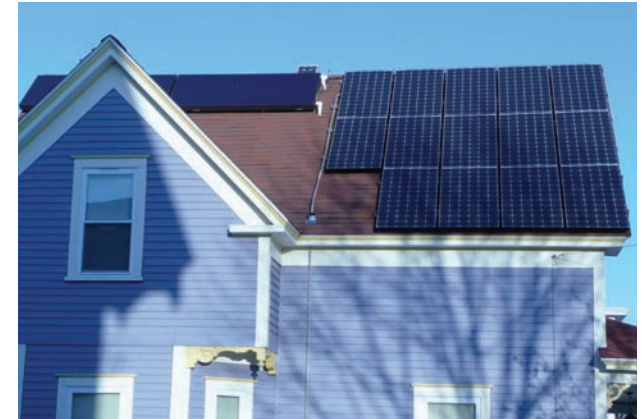
Photovoltaics, which convert solar radiation into direct-current electricity, and hot water panels on a home in Lowell Photo: DPD
