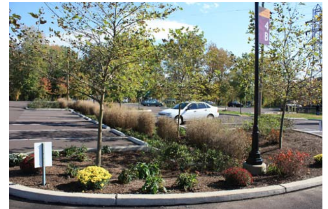
A parking lot incorporating bioretention practices Photo: Montgomery County Planning
