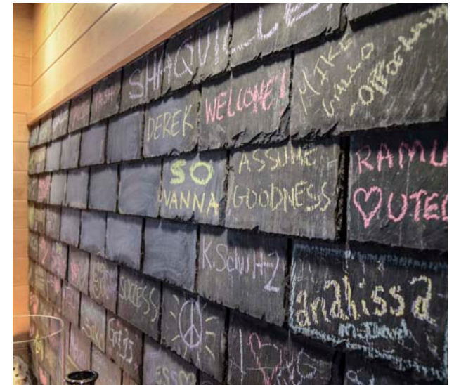
Recycling of old slate in UTEC’s award-winning retrofit, the oldest LEED Platinum building in the country. Photo: UTEC
