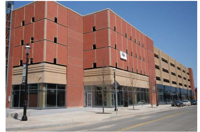
Edward Early garage street facade
