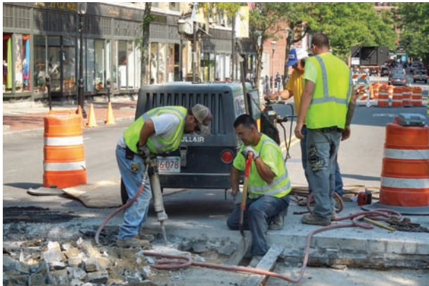
Central Street Repair
