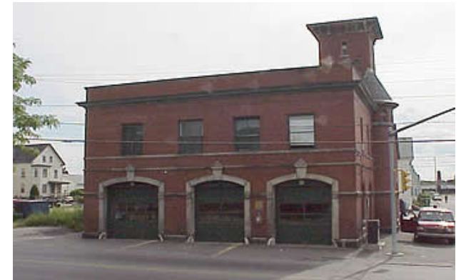
Gorham Street Firehouse. Photo: Lowell Fire Department
